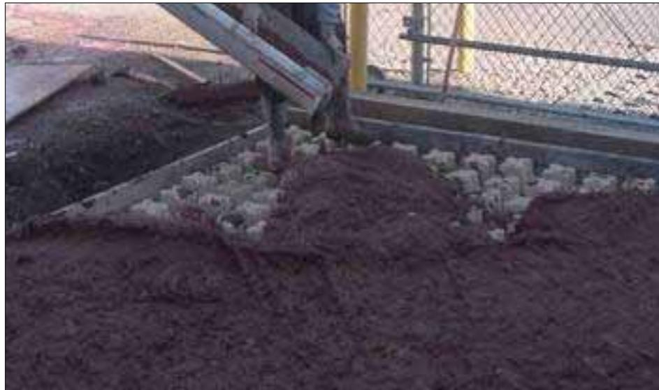
**46% Class F Fly Ash mix with 100% Reclaimed Crushed Concrete Aggregate**
